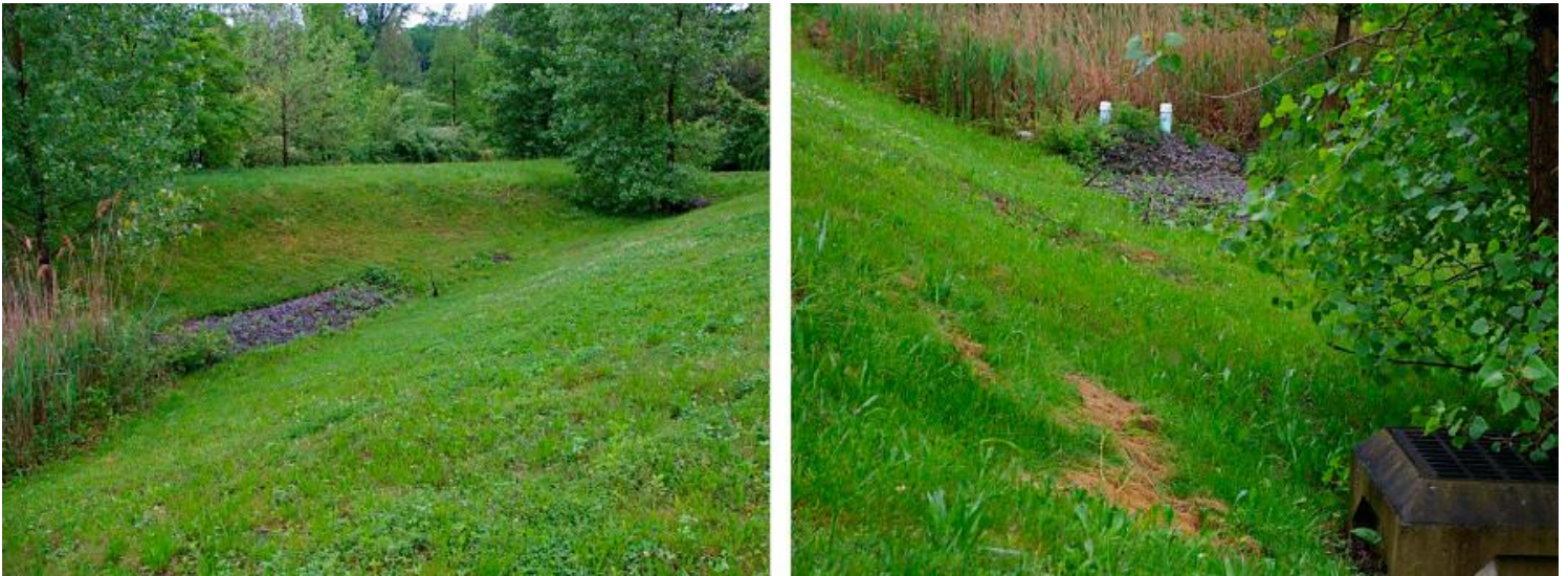
Grass filter strips discharging into water filtration basins. Source: Robert Alonzi.
